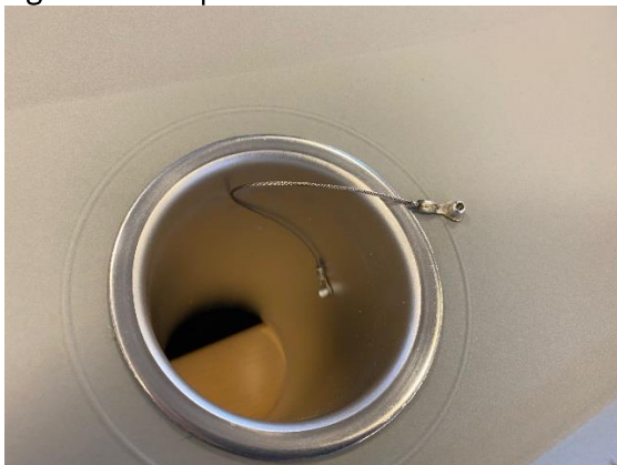
Figure 5: Example – internal bonding wire between the conductive hood and the aluminum tubing.
